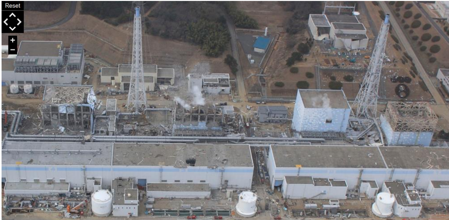
The four crippled reactors at Fukushima, picture from unmanned drone, 20 March. From right to left; reactors 1, 2, 3 and 4. Picture: AP/Air Photo Service.
